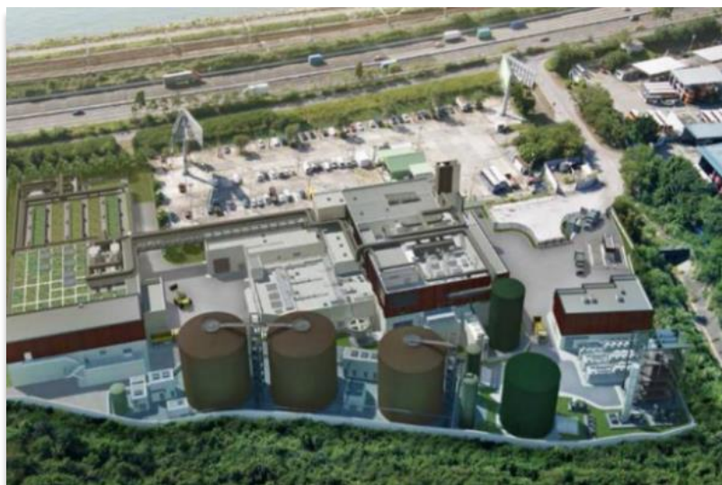
Organic Waste Treatment Facilities (OWTF) Phase 1, O.Park1
