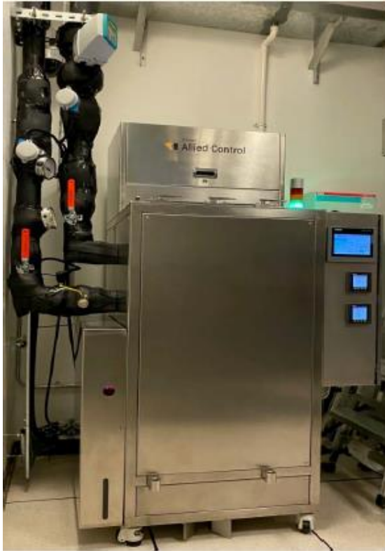
Immersion Cooling System for servers in Data Centre
