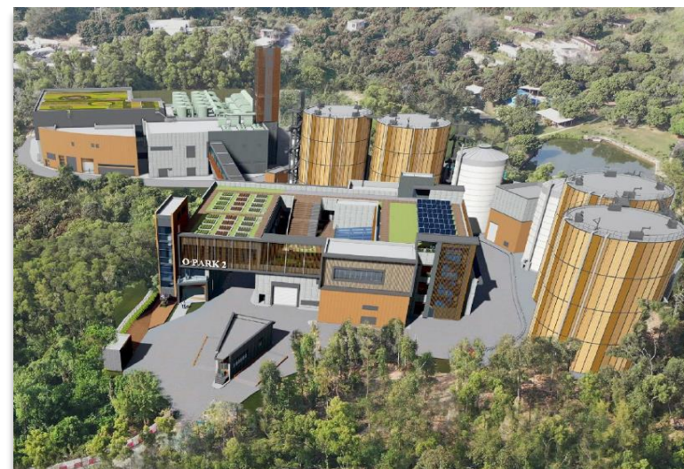
Organic Waste Treatment Facilities (OWTF) Phase 2, O.Park 2 (commissioned in Q1 2024)
