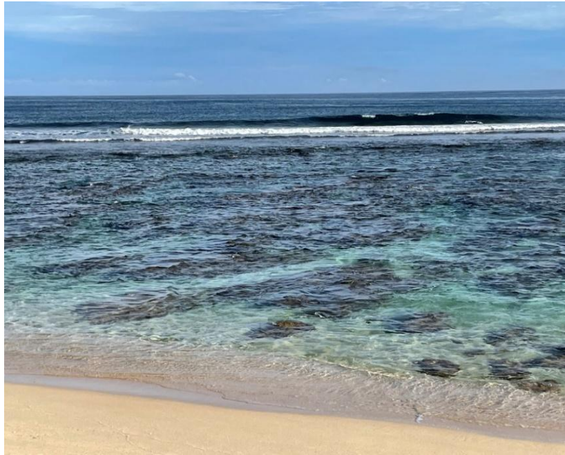
Exhibit 19. A live breakwater reef system.
