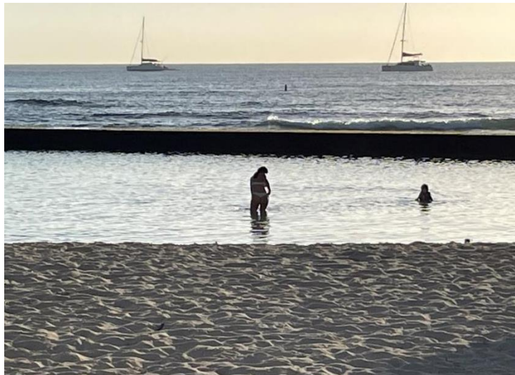
Exhibit 1. Seawalls that run offshore parallel to the beach reduce erosion caused by wind and tide driven waves. Waikiki Beach, Hawai‘i.
