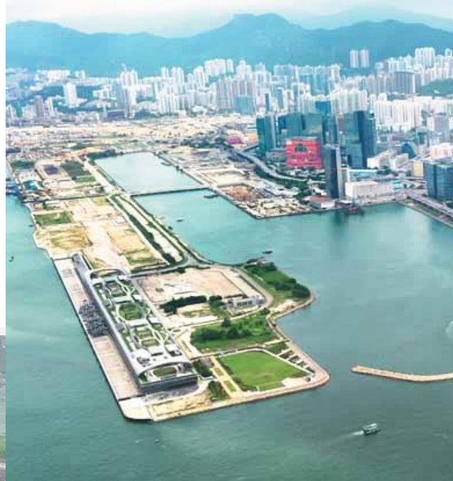
KTD under redevelopment
