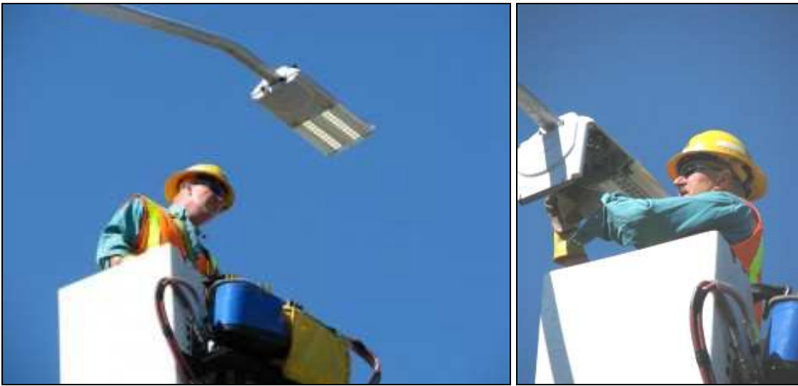
Figure 4.3 – Installation of LED Street Light in Seattle (Seattle City Light, 2011)
