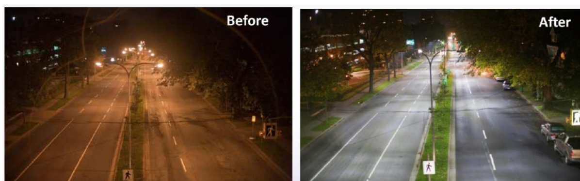
Figure 4.2 – Nova Scotia Street Lighting Demonstration Project - Before using High Pressure Sodium and After using LEDs (TAF, 2011)
